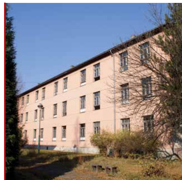
Under the ruling of the Federal Government a part of the former barracks 'Husein-kapetan Gradašćević' was allocated to the University of Tuzla.
