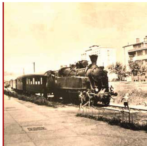
The construction of the 67-kilometer long Doboj –Simin Han Railway was completed in 1886.
