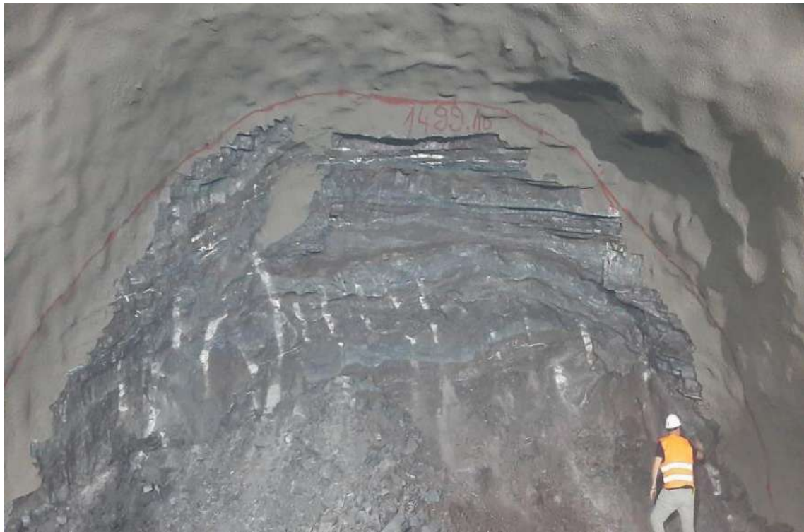
Figure 2. View of the work face, chainage 1+499.10 - left tunnel
