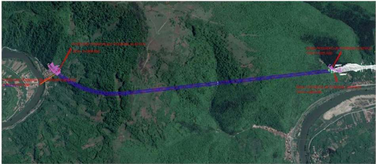
Figure 1. Geographical position of the Zenica tunnel on the Corridor Vc route
