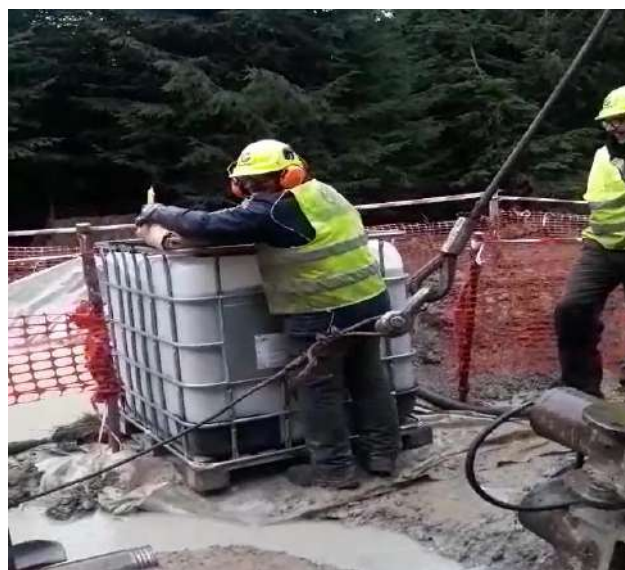
Image 5. Mixing bentonite in a 1000-liter container
