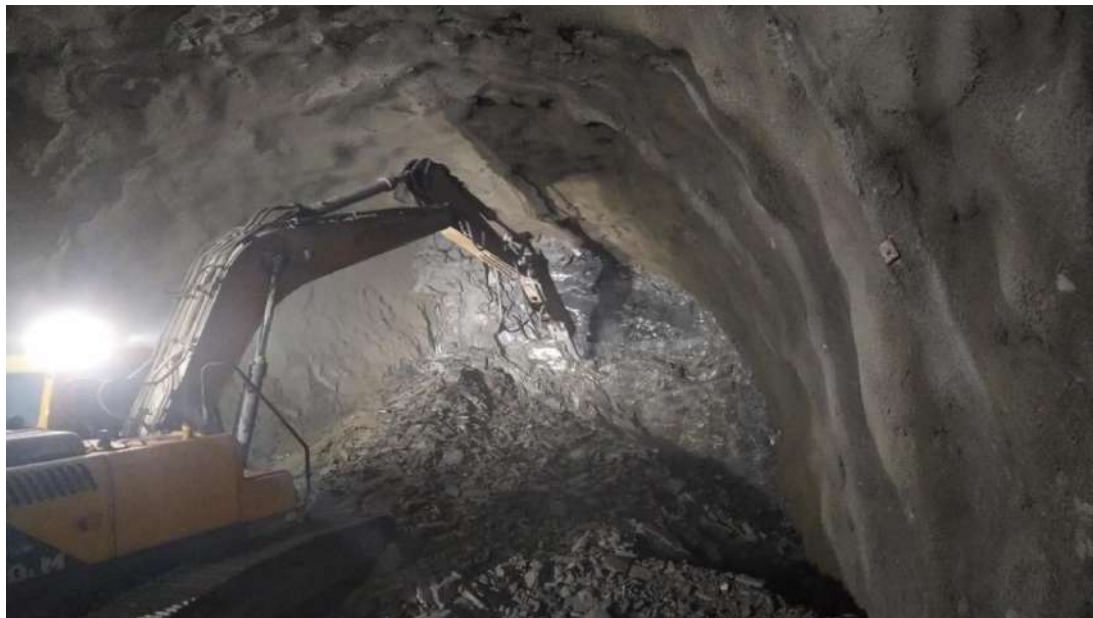
Figure 6. Machine excavation of full cross section in LTT at chainage 1+518.00 to 1+520
