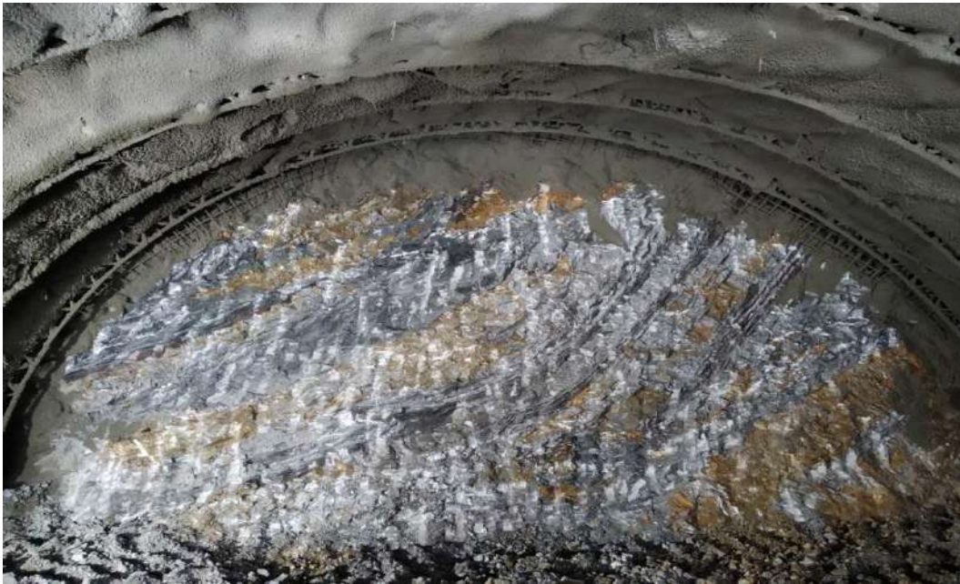
Figure 1. The head of the Zenica tunnel excavation
