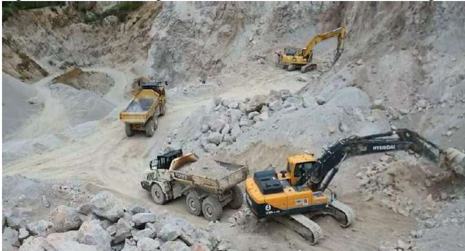
Figure 4. Loading of materials after blasting on the floor
