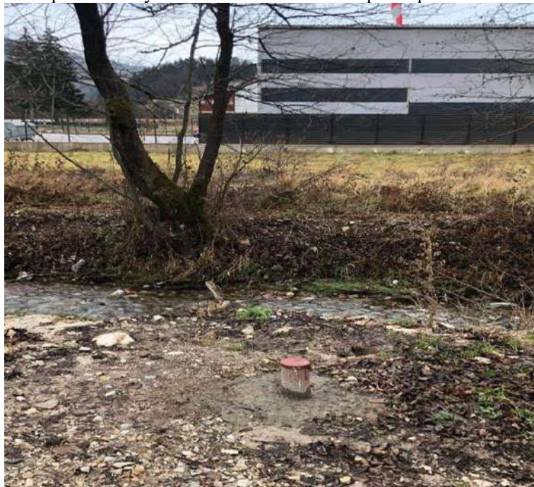
Figure 3. View of the built-in protected piezometer
